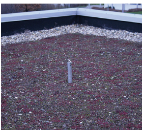
ParaSave P1 Fall Protection – installed
